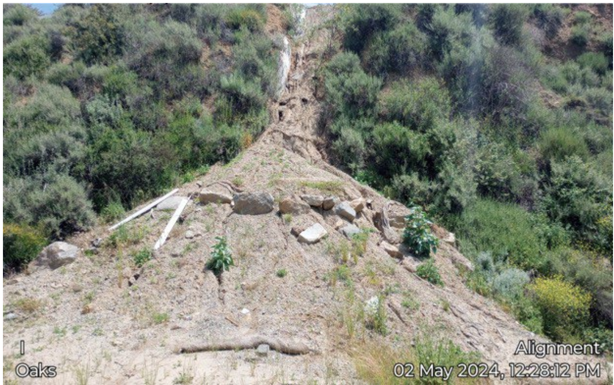
Photo 8. Southern drainage alignment, looking east to terminus.
